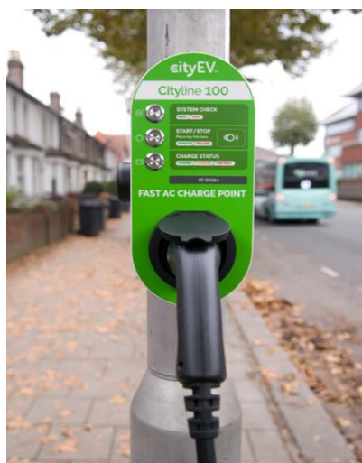
Figure 3 – Lamp column EVCP 32
